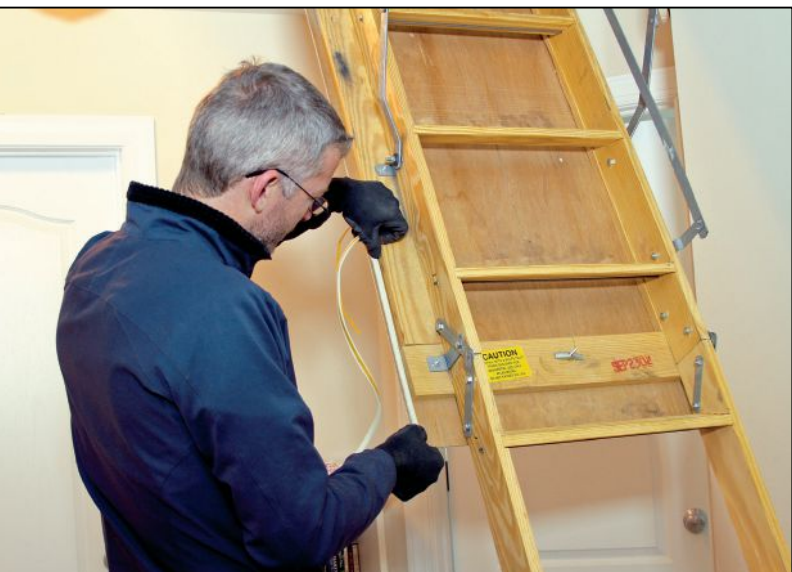
This standard attic hatch has been insulated and weather stripped to reduce energy waste. Photo source: EnergySmart Academy
