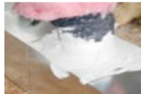
Apply mastic directly on the duct
