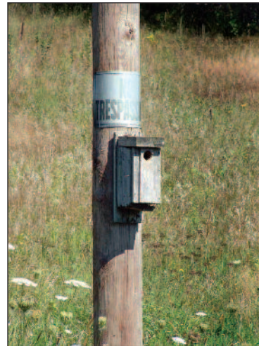
An illegal birdhouse perches on a utility pole below an equally illegal sign. Source: Allamakee Clayton Electric Cooperative
