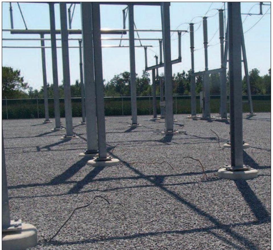
**Only small lengths of copper grounding lines remain in a substation after thieves stole the wires. The loss of grounding on electricity distribution infrastructure increases the risk of electrocution to anyone in the area. But with the price of scrap copper skyrocketing, burglars risk life and limb to score a quick buck.**
